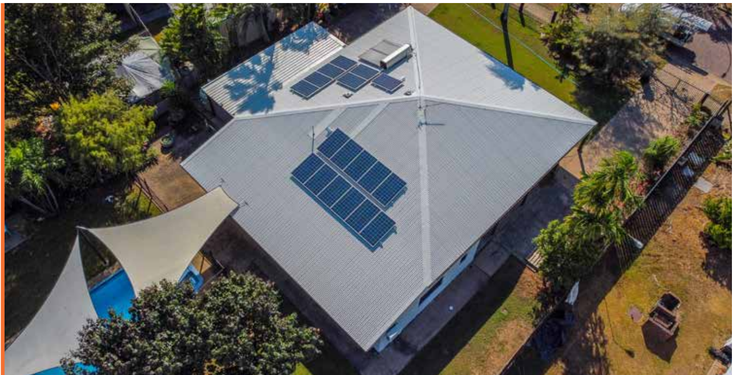
Koolpinyah Crescent - Re-roofing, insulation, skylight & whirly-bird
